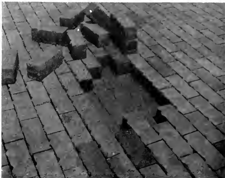
Fig. 3—Bricks removed from pavement.
